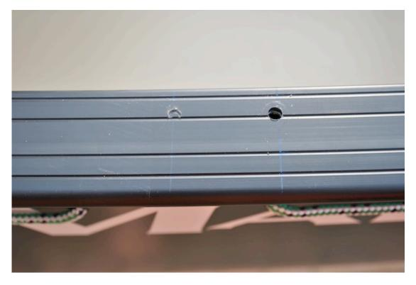
In the picture above a drilled hole can be clearly seen along side the mark created by screwing the bolt through the riser.
